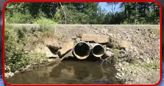
Figure 23. Pipe Culvert (USFW 2022)
